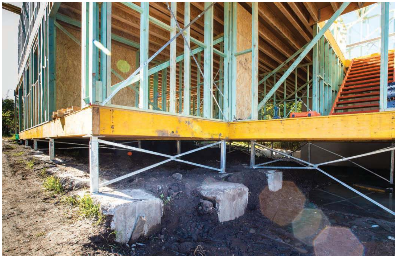
Figure 13 An example of galvanized steel posts being used in combination with a traditional timber frame and subfloor.
