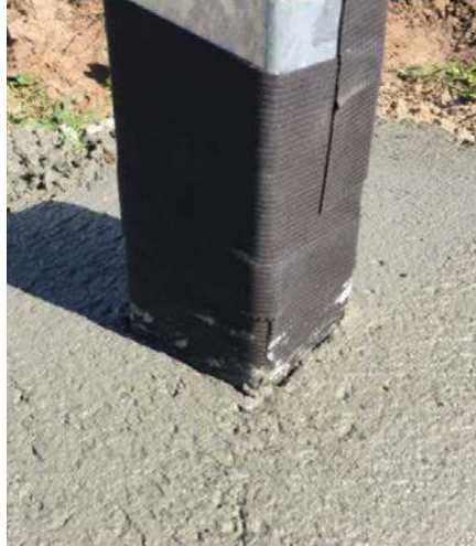
Figure 10 Denso Ultraseal tape wrapped around the base of a newly embedded post.
