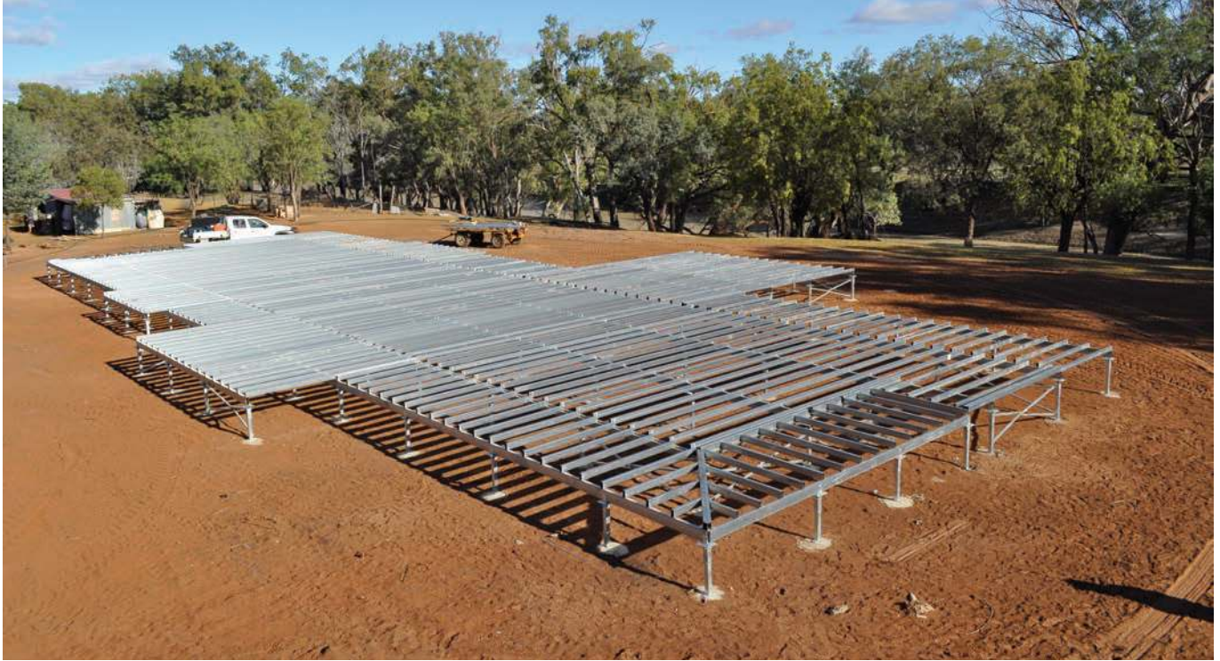
Figure 3 Batch hot dip galvanized structural steel posts in combination with a continuous galvanized sub-floor located in a BCA moderate zone (more than 1km from breaking surf).
