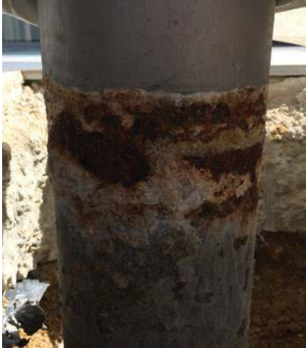
Figure 9 A galvanized post without additional protection at the steel and concrete interface showing accelerated corrosion which has reduced the overall durability of the structure. Note the galvanized coating above the ground remains in excellent condition.
