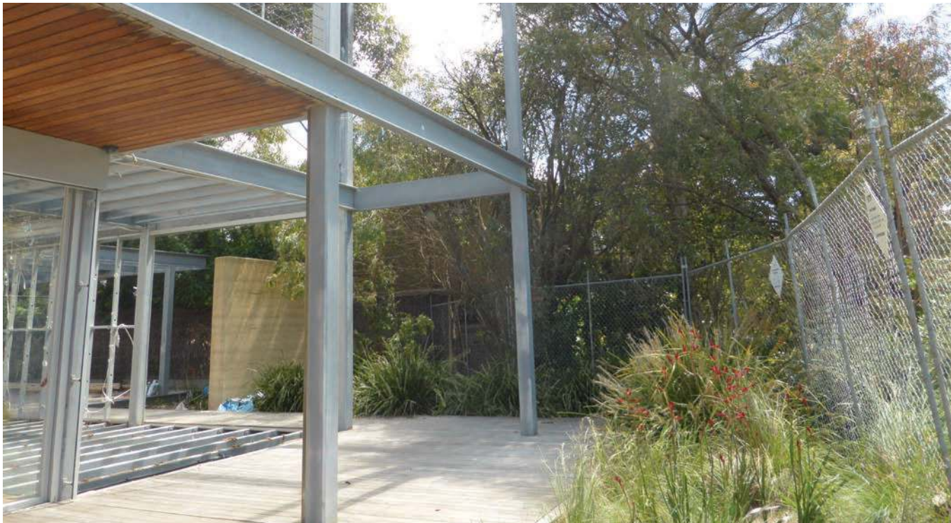
Figure 5 The galvanized structural steel members (verandah posts and edge members) have good access and would be expected to provide structural support with regular maintenance of the galvanized coating for 50 years in moderate locations, while regular maintenance, plus repairs to the galvanized coating would be expected during the life of the building in severe environments.
