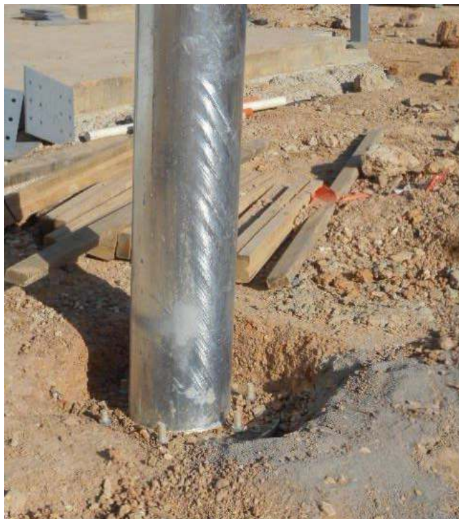
Figure 7 This large post bolted to a concrete pad will finish below the ground level and will be at risk of collar corrosion reducing the durability of the structure.
