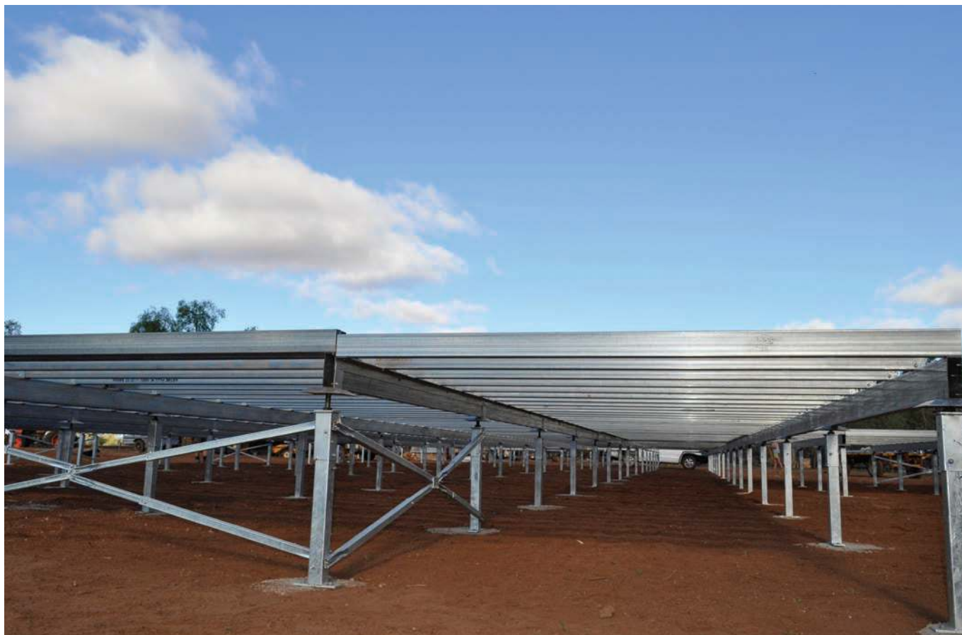
Figure 12 A galvanized steel subfloor (with inbuilt ant caps) where the hot dip galvanized posts bolted down onto elevated concrete pads.
