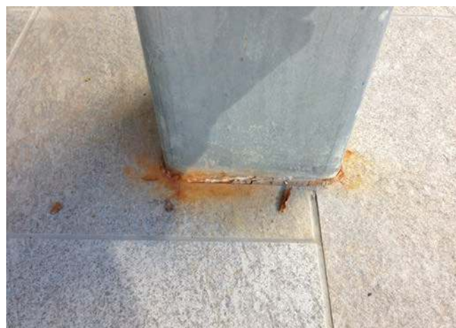
Figure 4 A verandah post embedded into a tiled floor in a wet area. Water has seeped into the gap between the tile and the steel through capillary action, leading to accelerated corrosion and early failure. This is a design defect where separation of the water from the steel was not considered.
