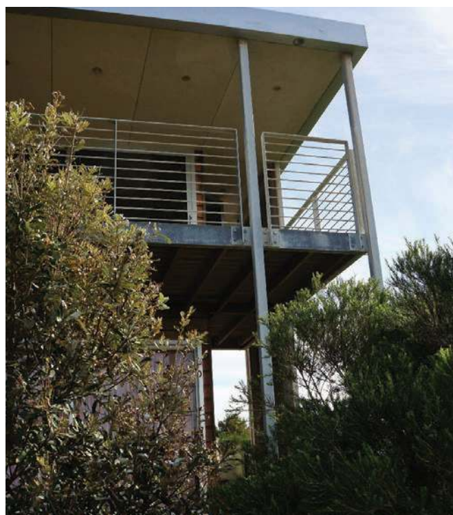
Figure 6 The top floor of this house overlooking the ocean is enclosed, while the underside of the balcony is open providing for different micro-environments in the same house. In addition, the plants may offer sheltering from rain but not wind-blown salt, leading to a complex corrosion design.
