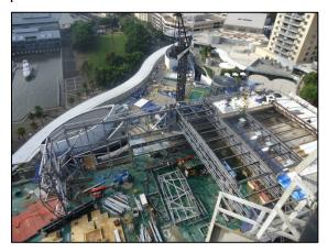
Effectively the steel frame is sandwiched between the interior soundproof walls of the MUEF and the attractive external stainless-steel and glass façade. In such a structure, the asset owner needed a guarantee that minimal or no-maintenance would be required for an extended period. The durable nature of the HDG coating ensures it will exceed the warranty period providing a maintenance-free service for at least 10 years.
