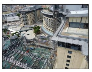
The MUEF is a 40 by 60 metre complex geometric structure that utilises a 300-tonne galvanized steel frame to support internal walls and an external glass façade which is internally lit at night to spectacular effect.
