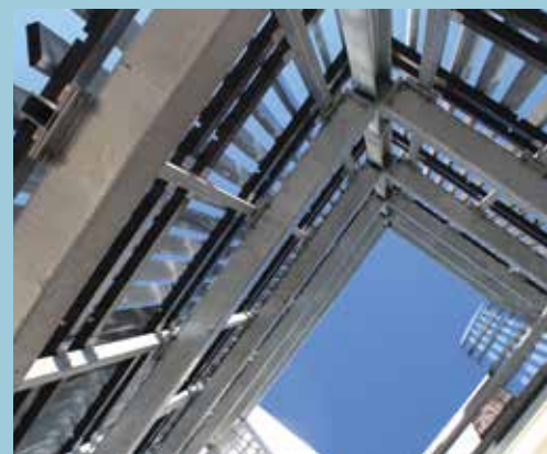
Austin Hospital Car Park, Melbourne
