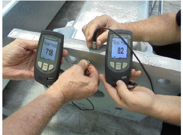
FIGURE 4: Measurements showing significant variation in coating thickness on flame-cut edge
