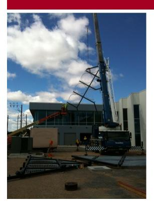
As an architectural feature of the steel facade, it was imperative the finish was consistent, requiring selection of domestic equivalent steel chemistry from the same steel supplier. With a "meccano" type construction of the facade required in order to bring the various components together, very tight tolerances were involved. This was reduced to several millimetres to accommodate a number of the in-fill panels, which can be hydraulically rotated. This, of course,
