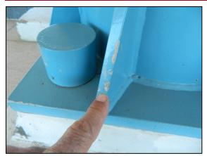
stainless steel corrosion may well be related to incorrect specification of the material.
