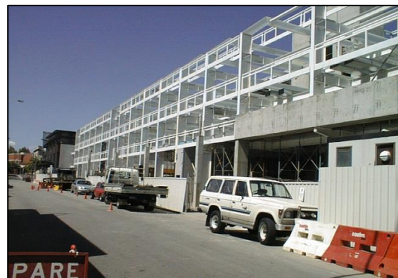
Figure 2: The structural frame of the car park during construction.
