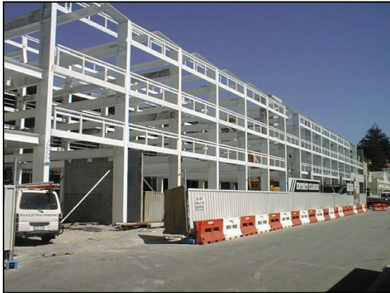
Figure 1: The Collie Street Car Park during construction in 2003.
